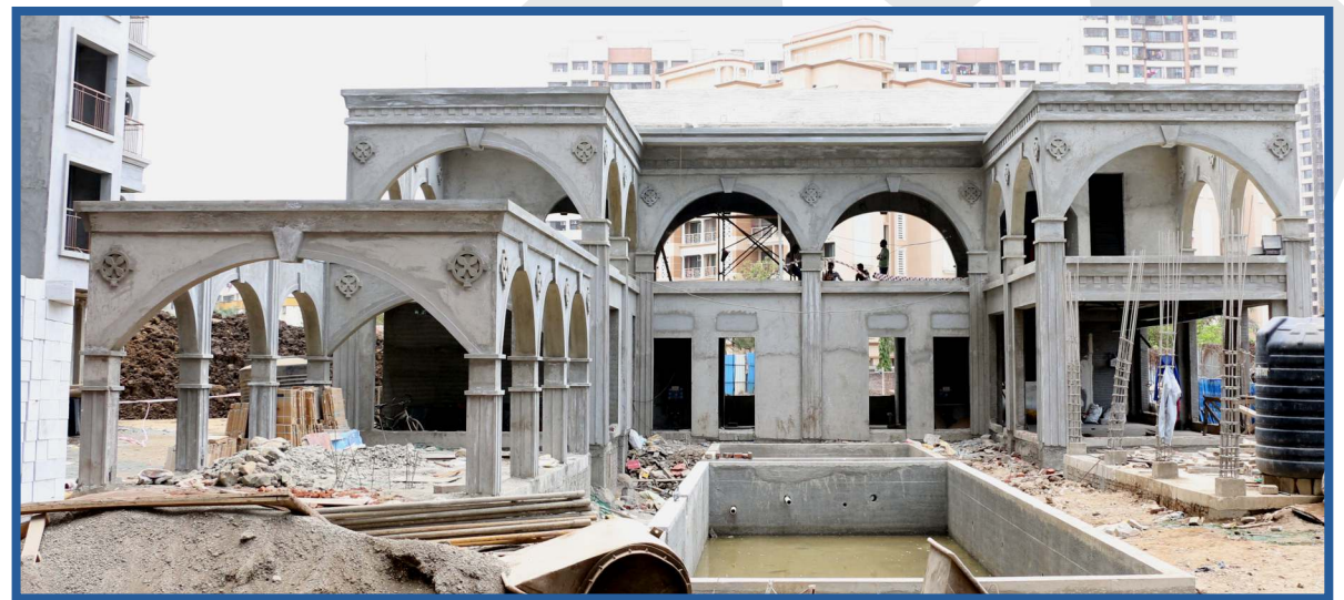
Club House Work In Progress
